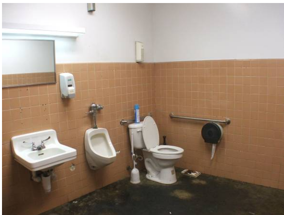
View of Rest Room
