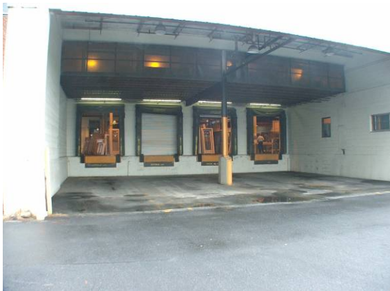
View of Loading Area
