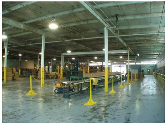
View of Staging Area
