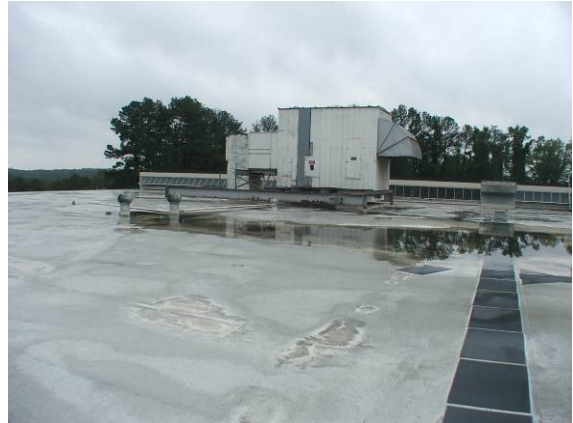
View of Roof
